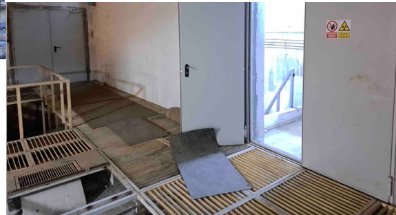
Entrance to the "secret" room (refurbished)
